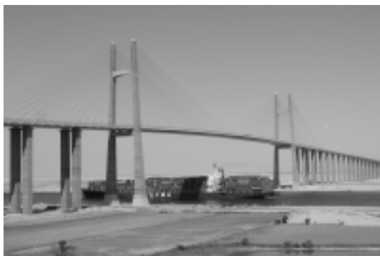
Photo 1 Suez Canal Bridge in Egypt (2001) 3-span continuous cable-stayed bridge (Total length : 730m, main span length : 404m)
